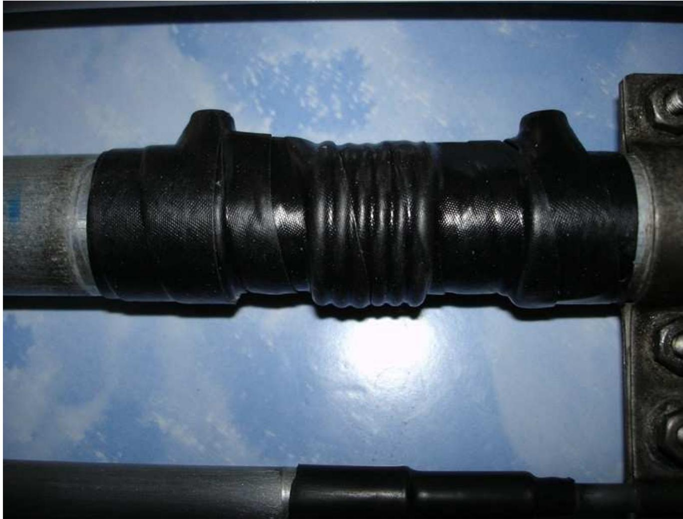
Application on 15 meter coil. Ensure that Alu tube must be sealed to the epoxy one
